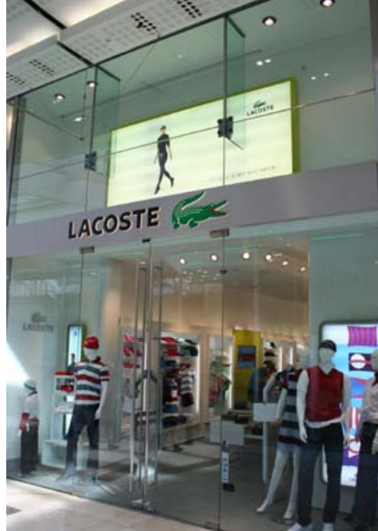
2. pushed through letters, internally illuminated
